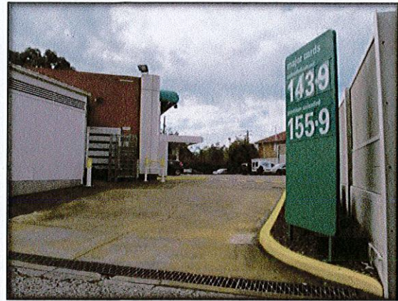
Figure 2.8: BP service station cross connection
